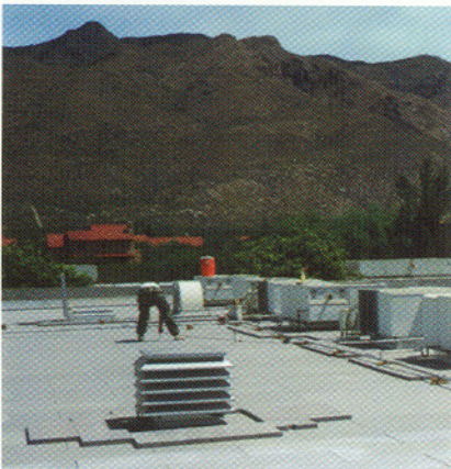
Emily Grey Jr. High School in Tucson, Arizona. Lightguard systems protect the membrane from maintenance traffic as well as vandals.
