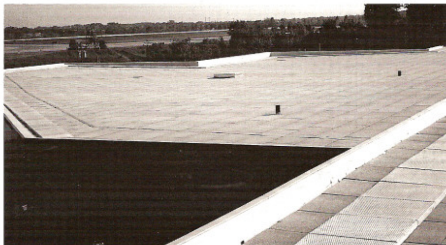
Husky Injection Molding in Buffalo, New York, used a T.Clear Protected Membrane Roof System with Heavyguard® Ballasted Roof Insulation to protect their building from the noise of nearby Greater Buffalo International Airport.
